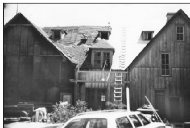
Roof repair in 1981 - Photo By Ray Padgett
